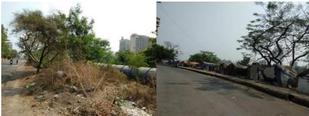
Figure 6. Encroachment in buffer space
