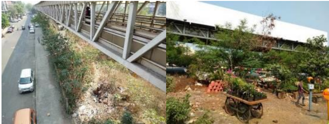
Figure 4. Encroachment below Skywalk
