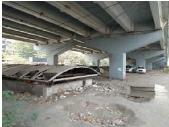
Figure 10. Area under flyover
