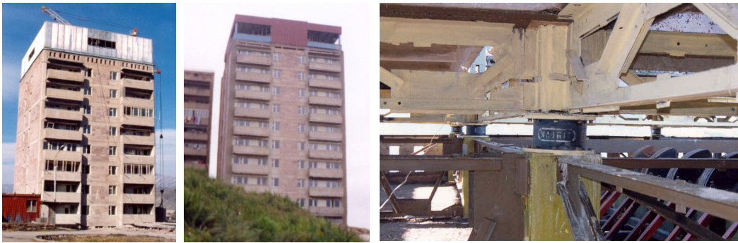
Figure 2. Steel rigid trusses constructed on the top of 9-story building and at the bottom of AIUF providing its reliable connection with the building by LRBs
